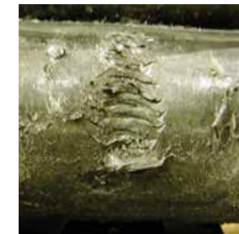
Minor cable damage caused by thread contact
